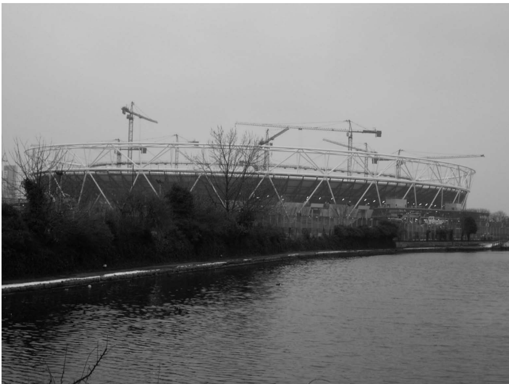
Figure 4.3 London main Olympic Stadium under construction in 2010.
