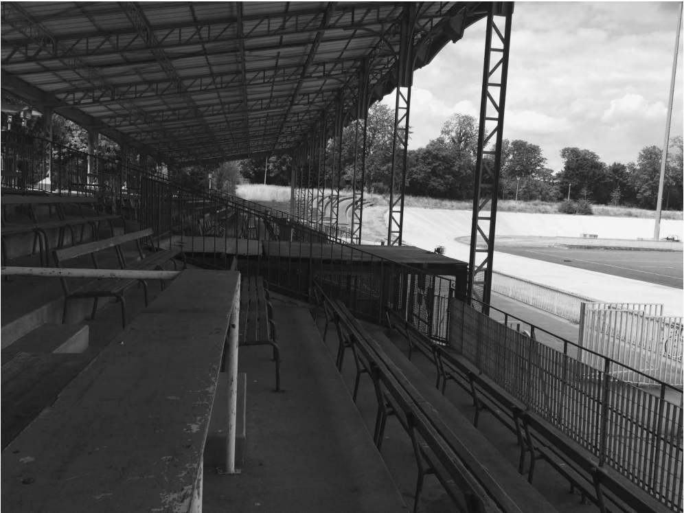
Figure 2.1 Municipal Velodrome, as it was in 2019. A charming stadium, with an illustrious history, on the edge of woodland.
